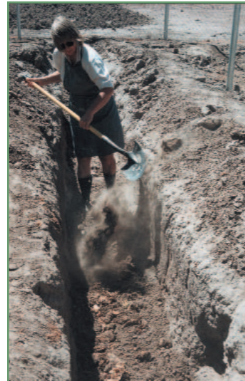
Trenching method at ASDB.
